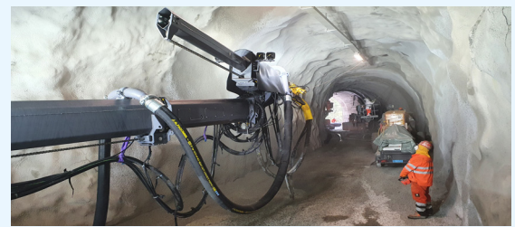
Shotcrete - Barmasse Tunnel
